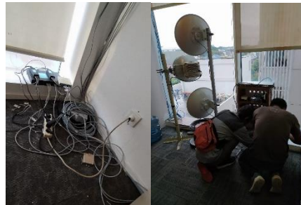
Gambar 5: Pemasangan Radio Antenna di Tower C
